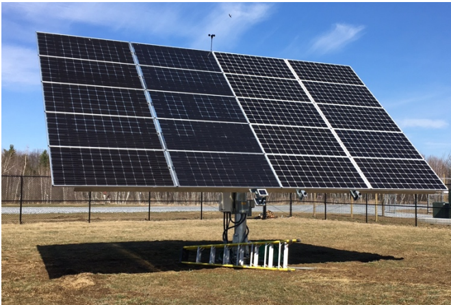
Fig. 1. Bifacial Tracker Two: 72-cell bifacial modules populate the left half; 72-cell monofacials are on the right. EETS reference cells and tracking error monitors are visible on the lower edge.
